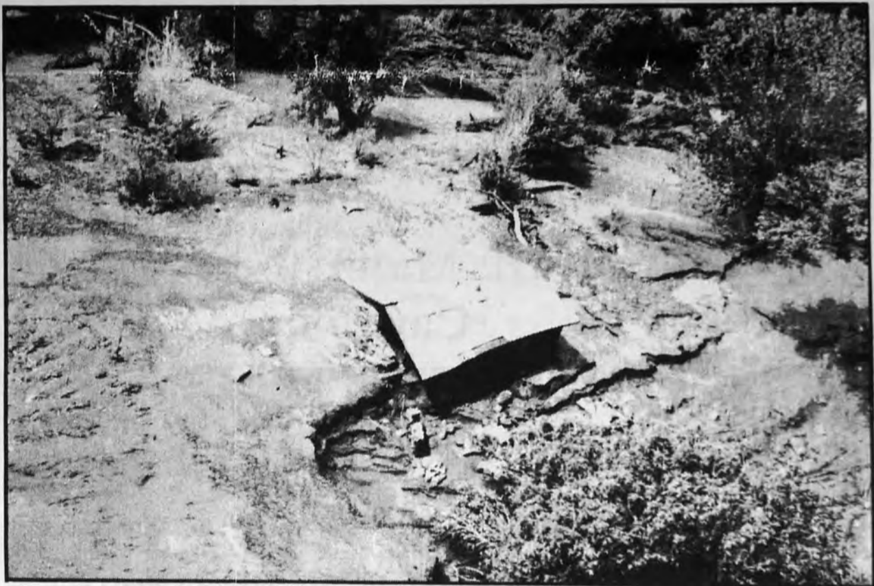
A Labor Day Flood at the Havasupai Indian Village, located downstream from Grand Canyon National Park, resulted in millions of dollars in damage to the village.
