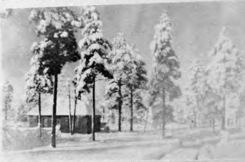
Cameron's Green house. The first schoolhouse at Grand Canyon
